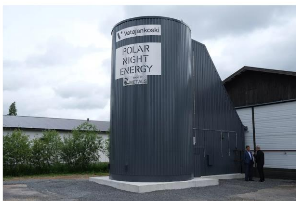
The sand inside the silo at Vatajankoski power plant in Kankaanpää can store heat at around 500C for several months. - Polar Night Energy
